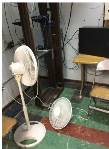
Exhibit 5B-11 Current Server Room Environmental Controls
